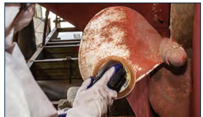
Removing old antifouling and sanding with power sander.
