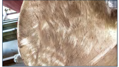
Close up of the clean surface ready for metal primer.
